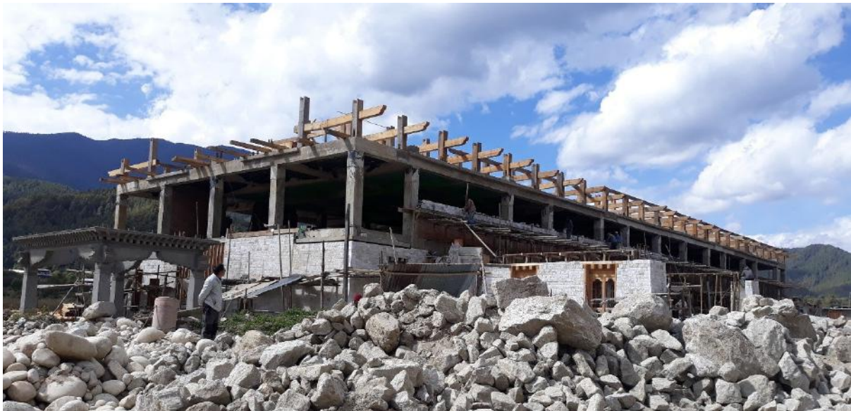
Figure 1: New Passenger Terminal Building construction at Bumthang Domestic Airport
