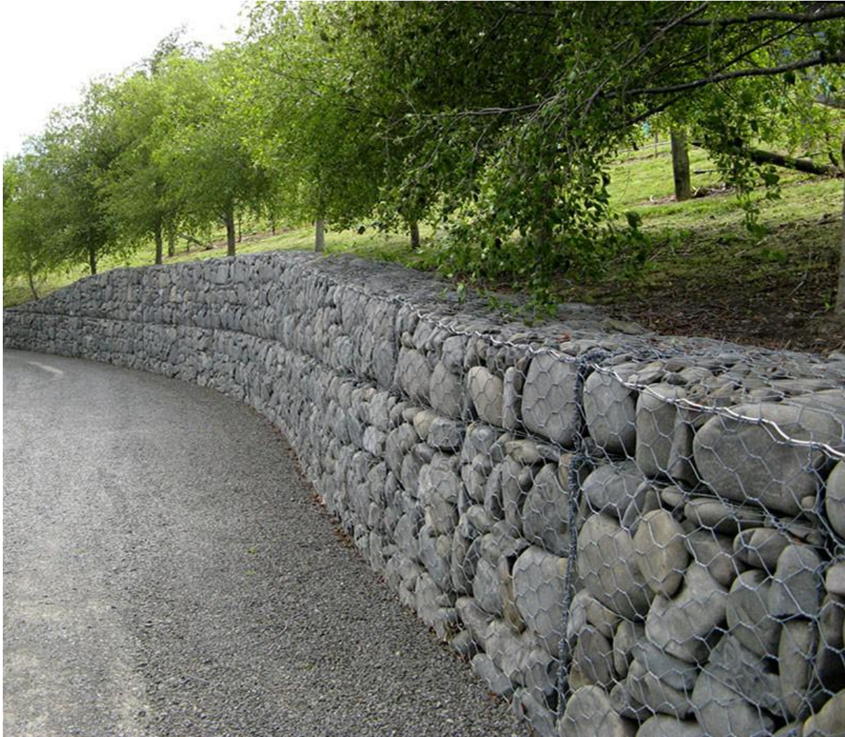
Figure 1: Sample gabion wall with plantation to stop soil erosion.
