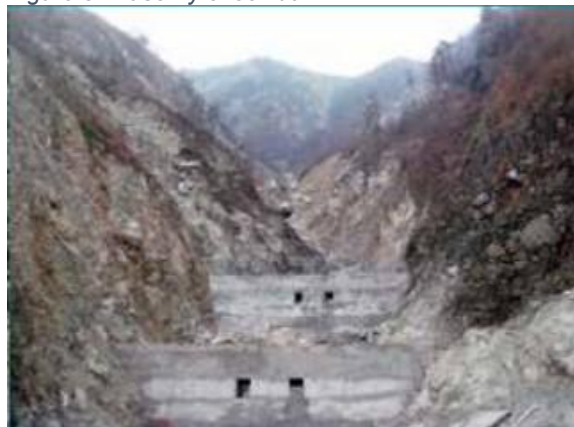
Figure 3: Masonry check dam
