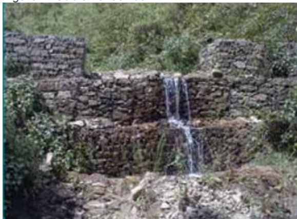
Figure 2: Gabion check dam
